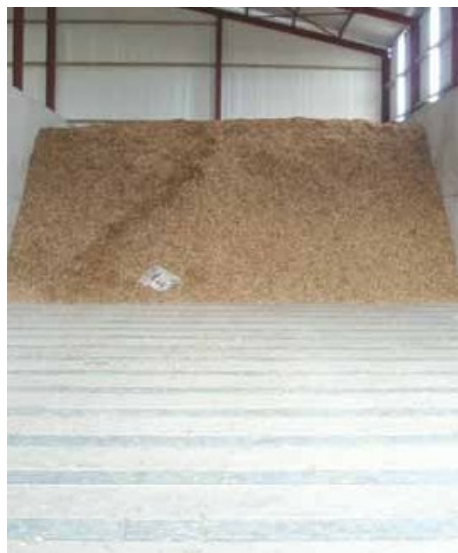
Figure 27: Ventilated chip or grain storage shed
