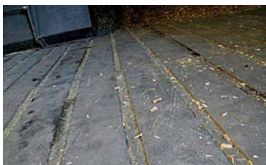
Figure 26: Detail of grain drying floor.(Sligo IT)
