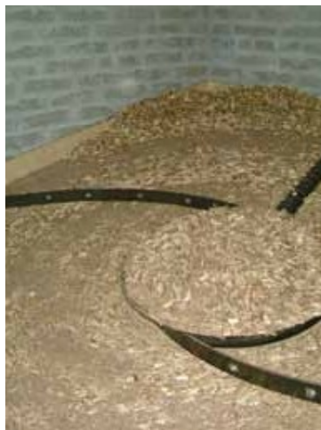
Figure 30: Wood chip store scraper system
