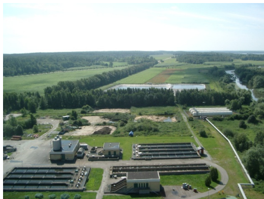
Figure 4.3: View of the Enköping municipal wastewater plant in Sweden, showing water storage ponds and willows used as vegetation filters
