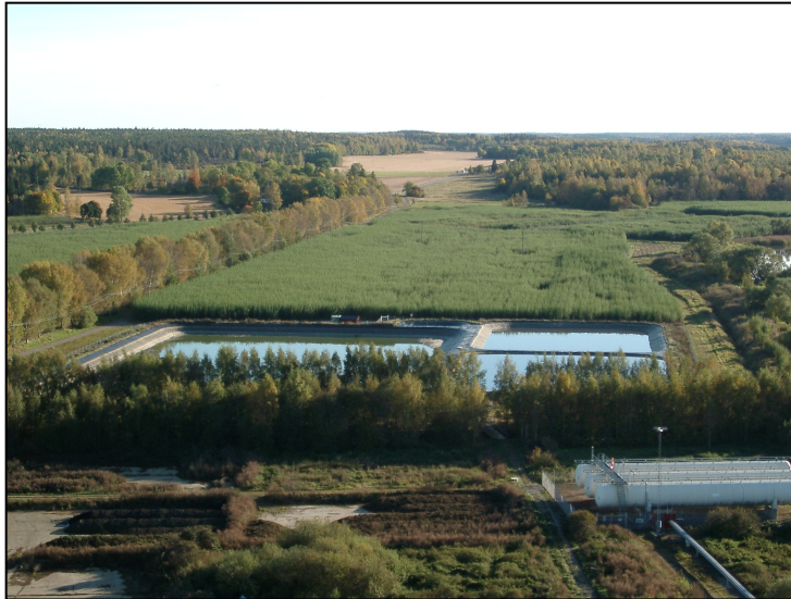
Figure 6. View of the Enköping municipal wastewater plant in Sweden, showing the water storage ponds and willows used as a vegetation filter. A 75 ha willow plantation treats and utilises decanted water from the dewatering of sewage sludge. The water contains approximately 25% of the N entering the wastewater treatment plant, but less than 1% of the water volume. By treating the water separately in the willow vegetation filter, instead of pumping it back into the treatment plant, the total N load is reduced by 25%. The biomass produced is used in the local district heating plant, contributing to the local supply of heat and electricity. Ash from the boiler is recycled back to the willow plantation. Courtesy: Per Aronsson, Swedish University of Agricultural Sciences, Sweden.
