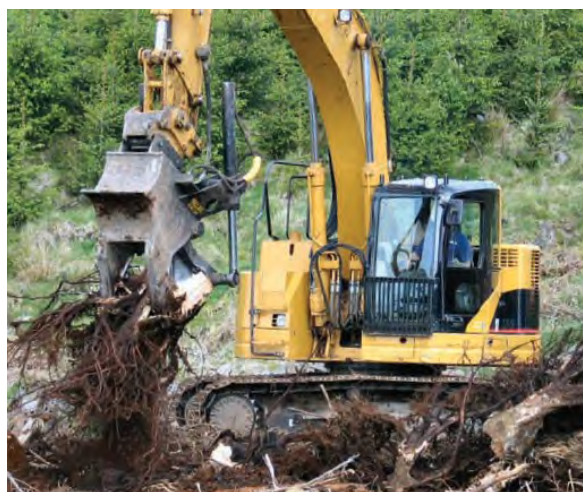
Figure 8. Excavating stumps (Moffat et al. 2011)
