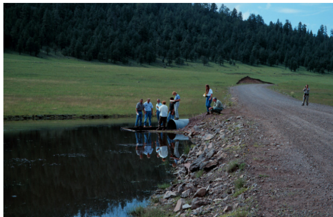
Figure 16. Storm runoff detention basin utilizing a constructed road fill, Cibola National Forest, New Mexico. (Photo by Roy Jemison).
