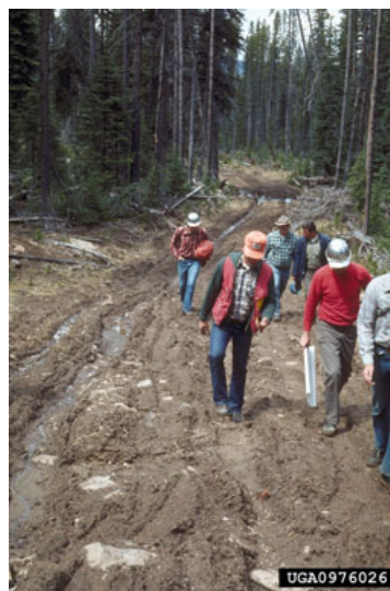
Figure 29. Rutting and eroded road segment causing sediment and water quality problems. (Photo by Dave Powell, USDA Forest Service, Bugwood.com).
