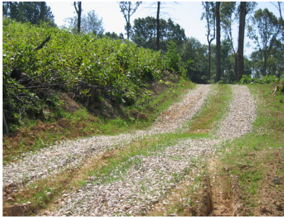
Figure 18. Broad-based dip in a forest road near South River, Virginia. (Photo by Matthew Yancey).
