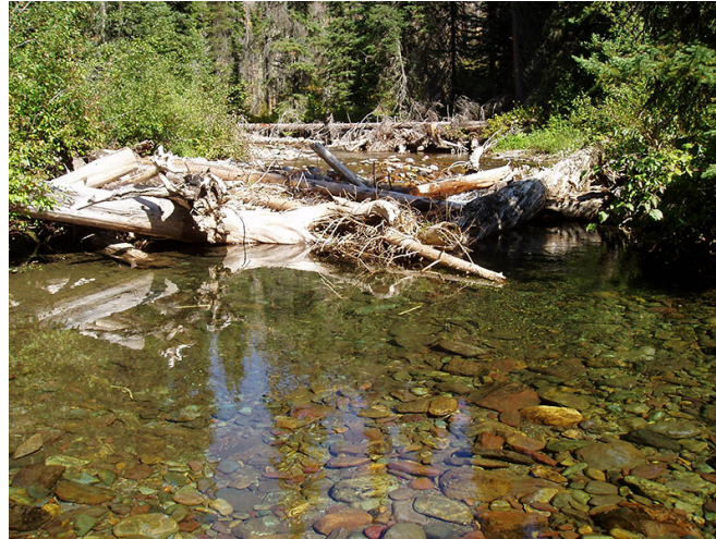
Figure 20. Woody debris left in a stream channel to improve fish habitat. (From River Design Group Inc.)
