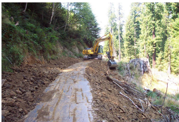
Figure 35. Sidecasting during road construction (Photo courtesy of Pacific Watershed Associates, http://www.pacificwatershed.com/projects/headwaters-forest-road-trail-conversion ).
