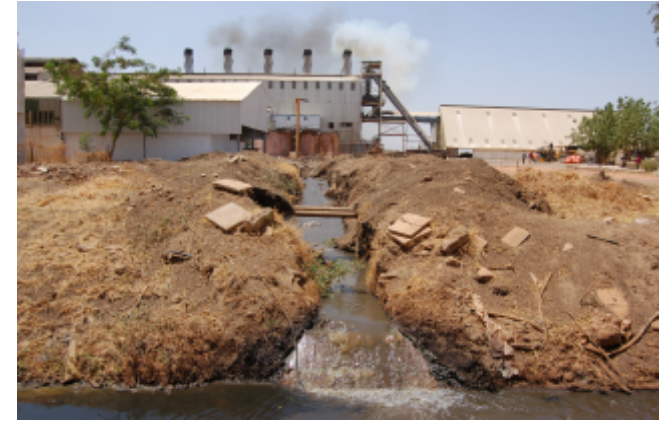
Absence of water treatment/sewage
